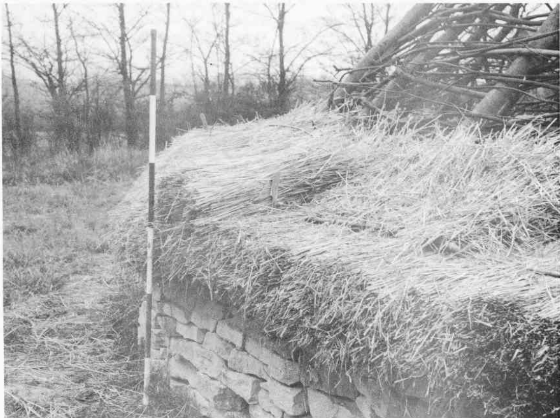
PL 10.9 The Conderton House eave; scale in feet
