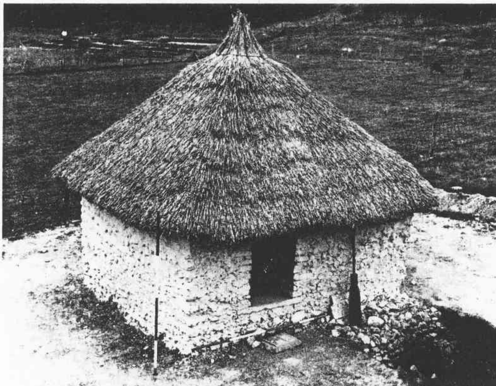
B. The completed structure with lime-washed walls, thatched roof and arched flue
