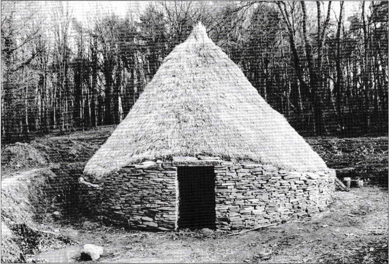
Plate 46 Museum of Welsh Life, St Fagans, Cardiff. Second Conderton construct, completed 1992. Photograph: Peter Reynolds
